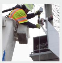
Lower winch line to the ground using a cordless drill with 5/8" socked adapter (adapter included).
