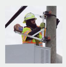
Position Handi-Hoist at the desired location on the pole and strap it securely using the 2 quick cinch safety straps.
