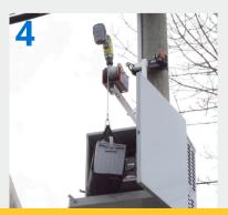
Using cordless drill in the forward direction, press the drill trigger to raise payload to the desired position.
