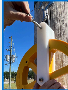
Re-insert retainer pin
