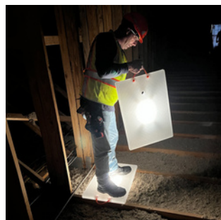
Position the next board at a comfortable distance. Step onto that board.
